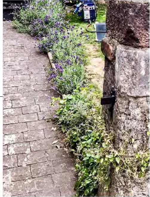
Existing concrete path with stamped paviour effect
